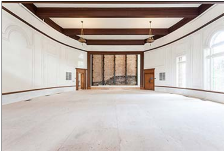
After the remodel, the 1925 Harvard Exit is now a Class A building inside a historic shell.
